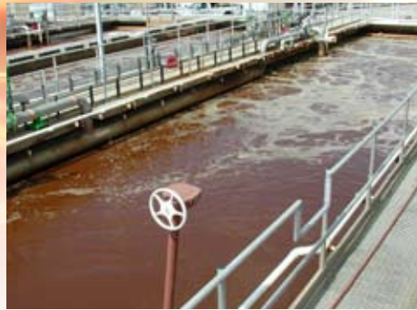
Phosphorus removal using iron salts
